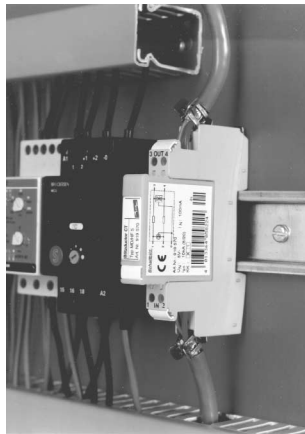
Figure B-3 Fine Protection in the cubicle Close to the First Bus Node
